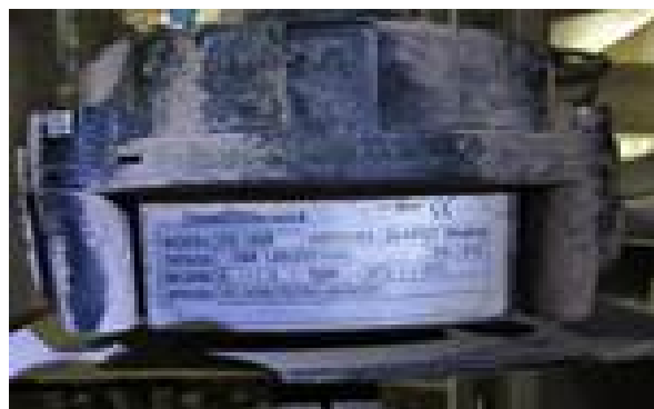
Ex d switchbox (Unreadable Marking)
