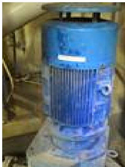
Ex Motors. (Lost Marking)
