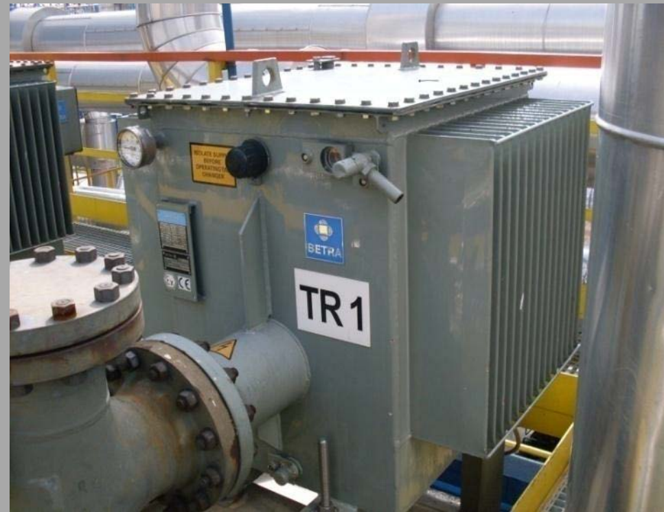
Transformer 100 kVA - oil immersion „o”
