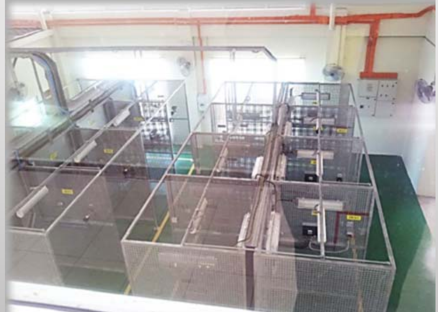
Performance assessment bays for the Unit Ex 003, Ex 007, Ex 008
